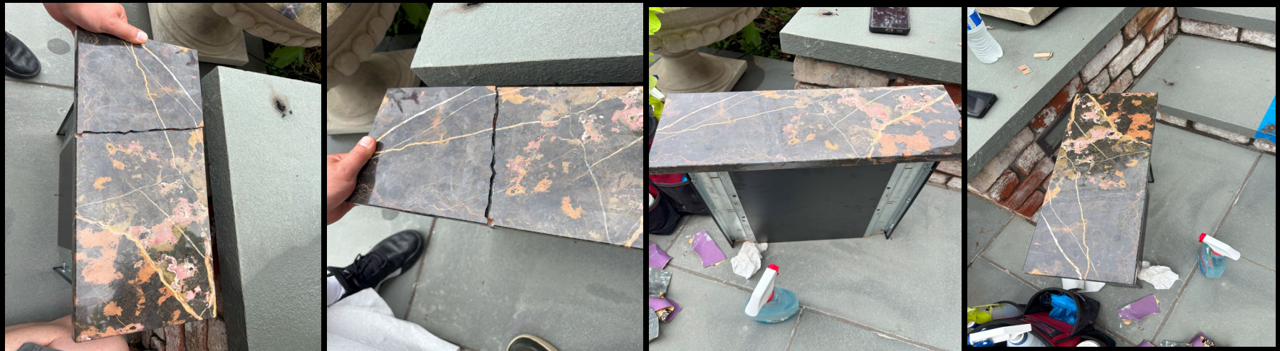
Aged marble drawer cracked (first two photos). Repaired and successfully color-matched (third and fourth)
