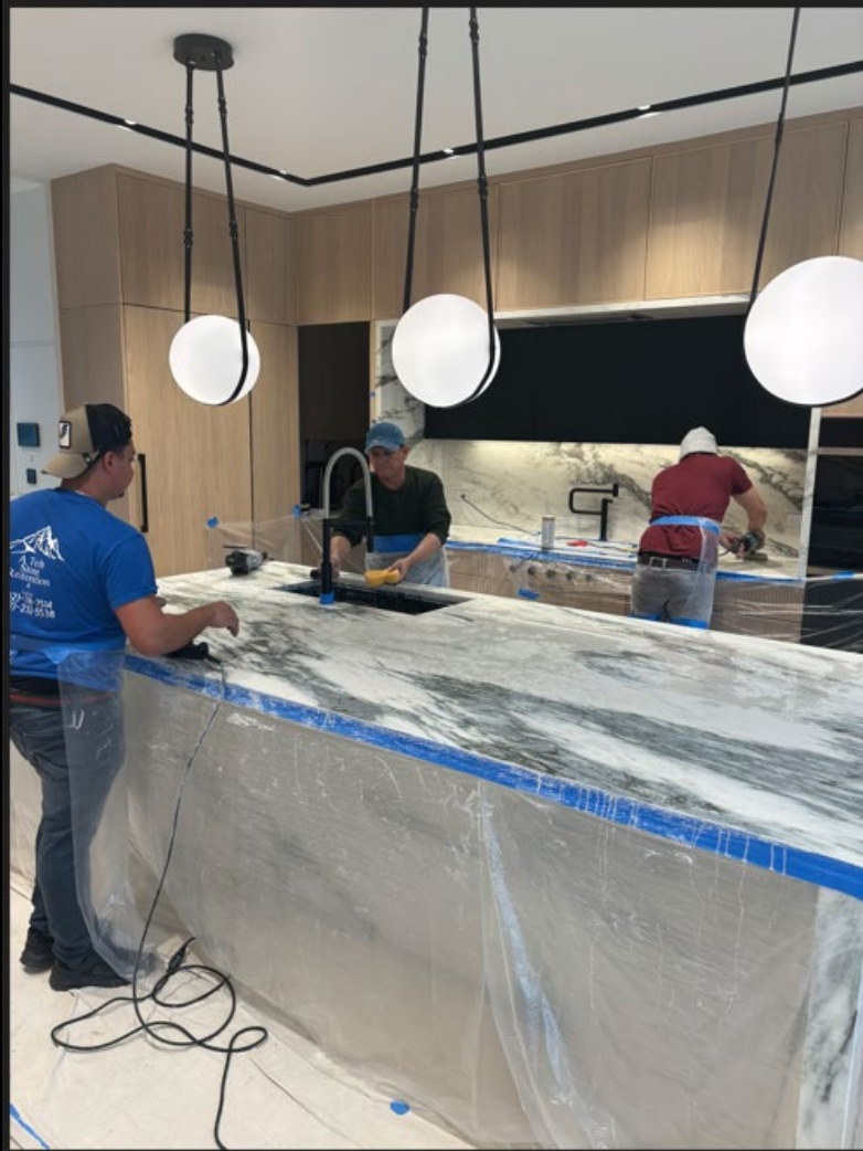
Resurfacing & Tuff Skin installed
