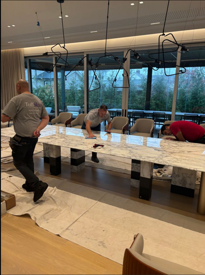
Resurfacing & Tuff Skin installed
