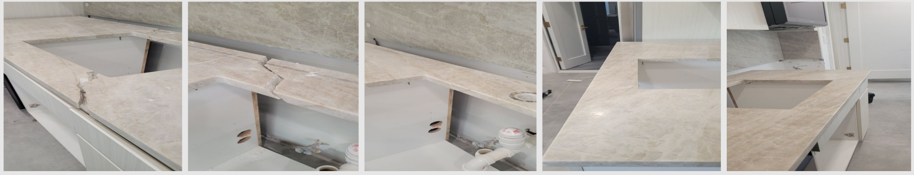
Quartzite cracked during plumbing work (first two photos). Repaired, color-matched, and refinished (last three)
